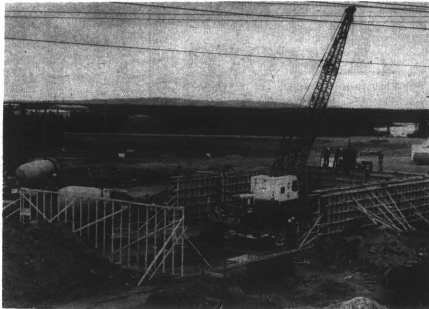
Work is progressing well on the new Union Hall Labrador City.
