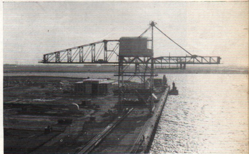
One of the giant loaders completed and in place.
