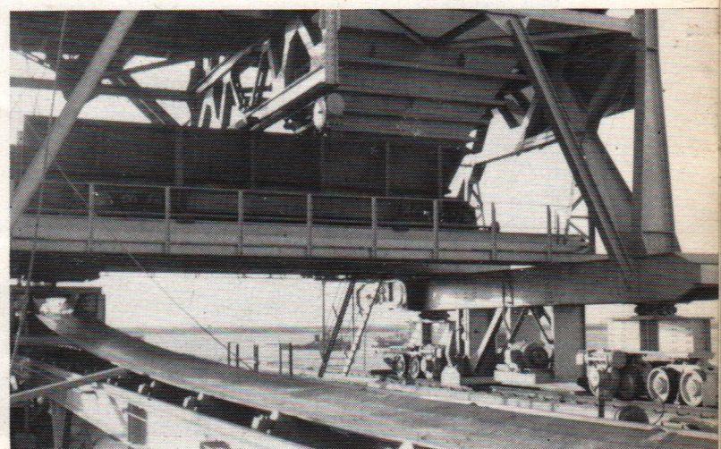
Belt and bin at the base of one of the loaders.
