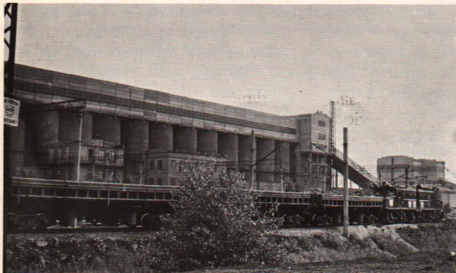
Storage silos for raw crushed taconite at the Krivoy Rog South Combine's concentrating plant are also reminiscent of Erie Mining Company.
