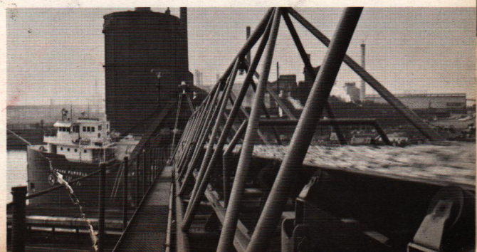
"Dock" at Muskegon, Michigan, consists of mooring spilings driven into water. Only a self-unloader can deliver bulk cargoes at this type of dock. Incoming cargo at Muskegon is primarily coal for utility plants.
