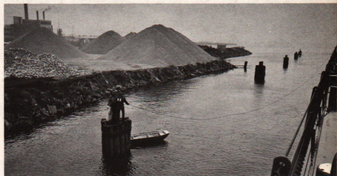
"Dock" at Muskegon, Michigan, consists of mooring spilings driven into water. Only a self-unloader can deliver bulk cargoes at this type of dock. Incoming cargo at Muskegon is primarily coal for utility plants.
