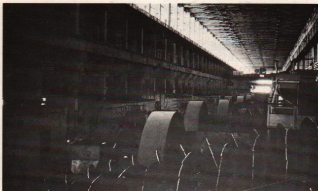
Taconite grinding mills inside the North Combine concentrating plant. Just as in our own installations, lighting is often a problem for photographers trying to show interiors of large bays. Soviet plants seem to be as well-lighted as our own, but varying light levels create exposure difficulties for the camera.
