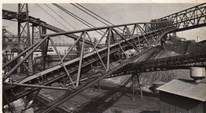
Boom can be placed very precisely, to unload cargo exactly where the customer wants it on his dock. Here, the Purnell unloads limestone at Chicago.
